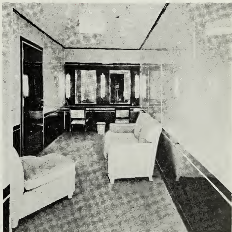
panels of plastic-finished Marlite were applied directly over the walls of the rough-textured plaster. Same material was used on the built-in vanity.
